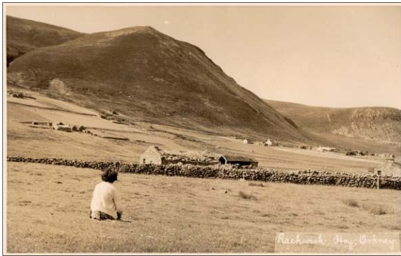
P11: Backdyke, looking north (HH233)
