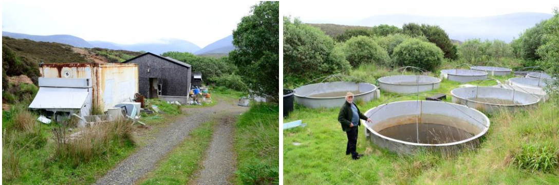
Figure 26. Fish farm (R96) hatchery (left) and tanks (right) prior to demolition.
